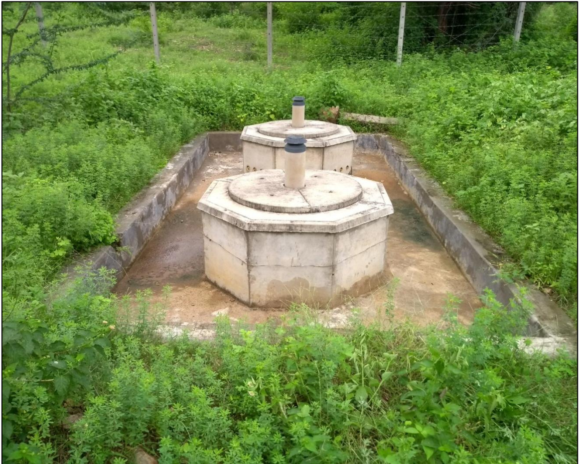
Scientifically developed Artificial Rainwater Harvesting Structure for recharge of Ground water resource
