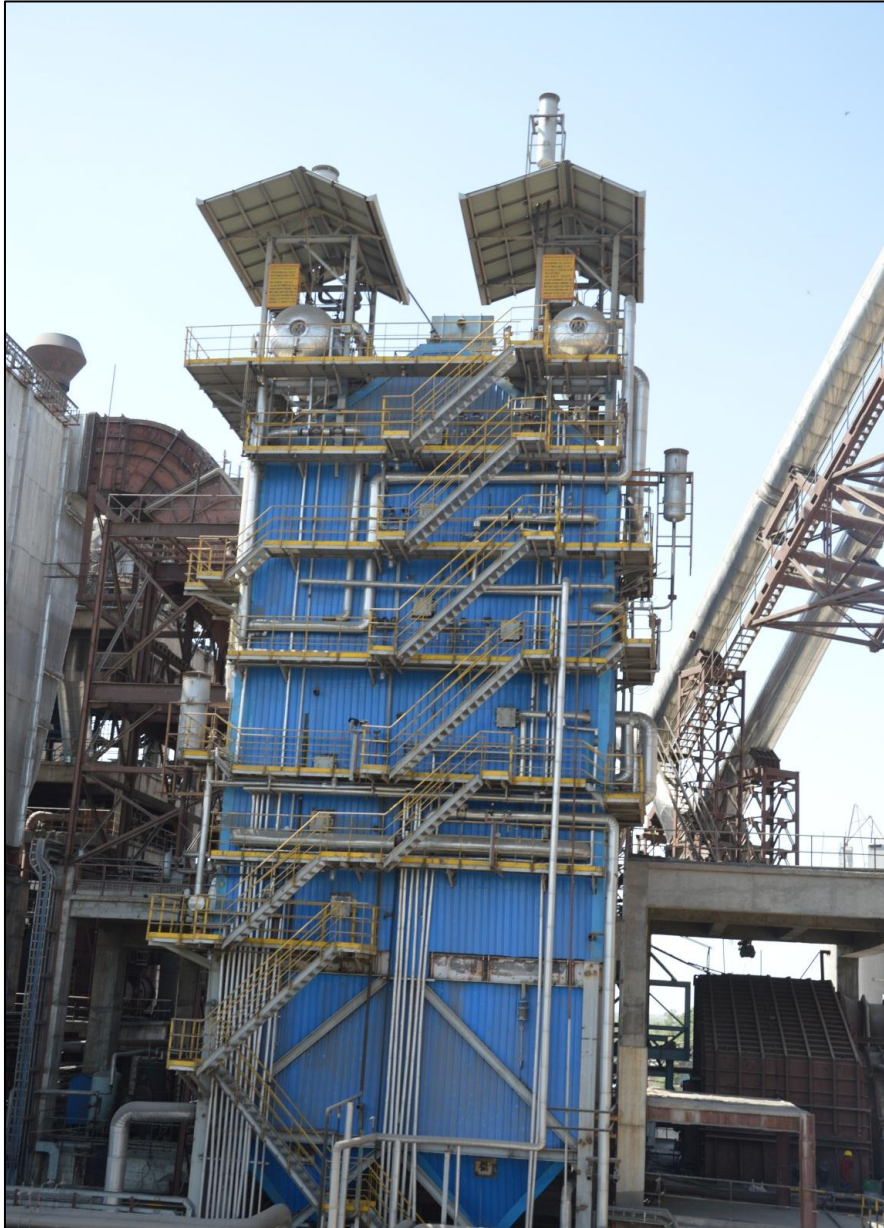
Waste heat recovery Power generating Boiler Unit
